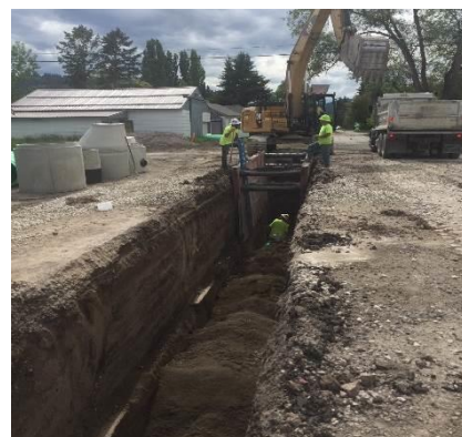
Figure 1: Schedule 1 Pipe Install
