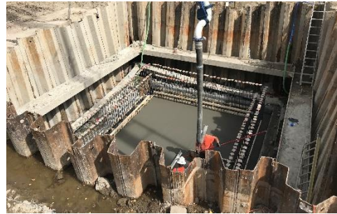
Figure 2: Schedule 3 Lift Station Base Pour
