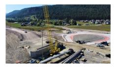
Construction of the Foys Lake Section of the Kalispell Bypass continues with 24 bridge beams for the overpass being set this week. The overpass will allow travelers to pass north-south over the east-west connecting teardrop roundabouts.
